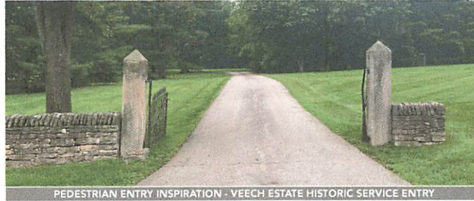
PEDESTRIAN ENTRY INSPIRATION - VEECH ESTATE HISTORIC SERVICE ENTRY
