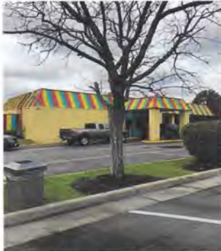
Post mortem on dead, thornless honey locust in Louisville: volcano mulch, planted too deeply, mechanical damage, poor soil and inadequate watering.
